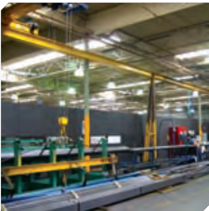
Clear and well-lit work areas allow the crane operator to clearly observe the load.
