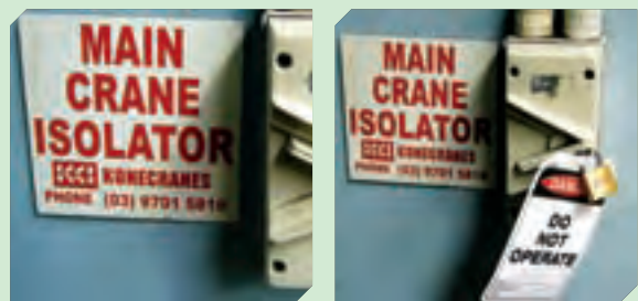
Main isolation switch isolated and locked in the 'OFF' position.
